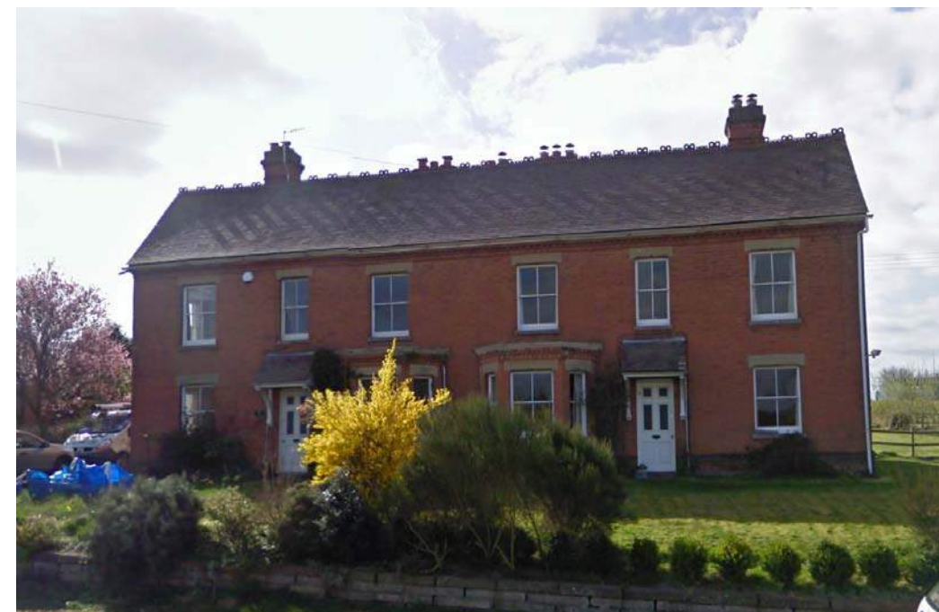
Photo 3: A pair of Victorian red brick semis on the A4104 frontage. Simple lines with use of bay windows, vertical proportions and gable roof with tile covering.
