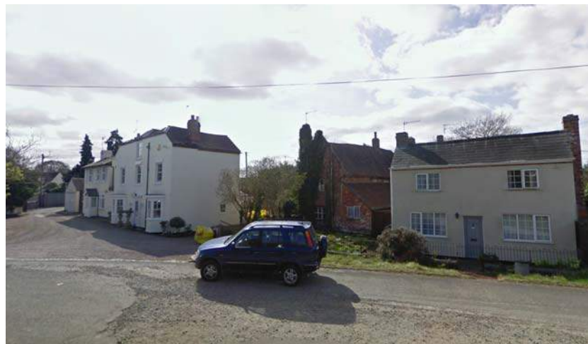
Photo 1: This 2-3 storey grouping on the A4104 frontage is mainly white rendered but also includes a red brick listed building.
